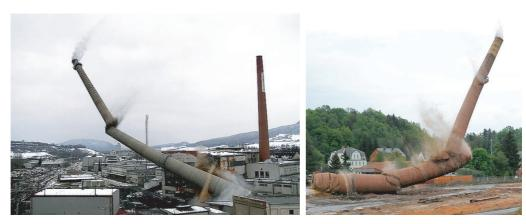
FIGURE 324 Falling brick chimneys – thus with limited stiffness – fall with a V shape (© John Glaser, Frank Siebner).
