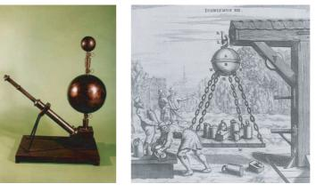
FIGURE 256 The pressure of air leads to surprisingly large forces, especially for large objects that enclose a vacuum. This was regularly demonstrated in the years from 1654 onwards by Otto von Guericke with the help of his so-called *Magdeburg hemispheres* and, above all, the various vacuum pumps that he invented (© Deutsche Post, Otto-von-Guericke-Gesellschaft, Deutsche Fotothek).
