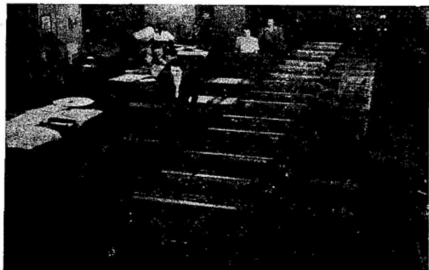
The differential analyzer, invented by Dr. Vannevar Bush of M.I.T. played an important part in servomechanism research. This photo shows G. E.'s version, with three operators at the input tables.
