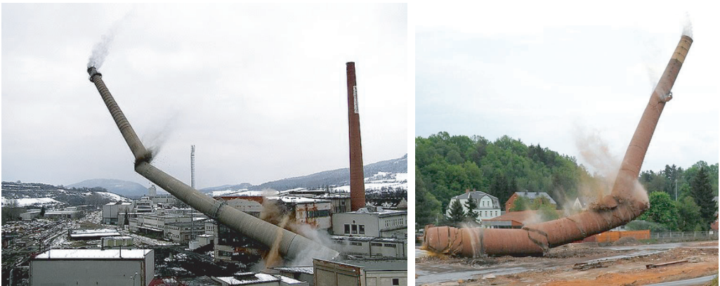
FIGURE 323 Falling brick chimneys – thus with limited stiffness – fall with a V shape (© John Glaser, Frank Siebner).
